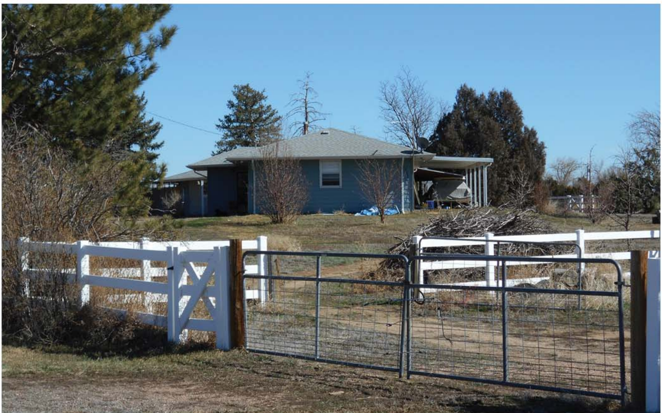
5AH3455_2: View southeast toward west side of house. Fencing separates the house and yard located on Parcel 118 from the animal enclosures and outbuildings located on Parcel 119 to the west.
