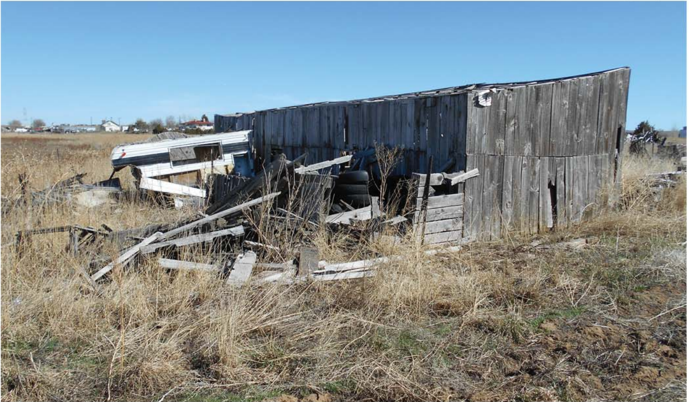
5AH3454_3: View southeast showing the north side of the building that is used for outdoor storage.
