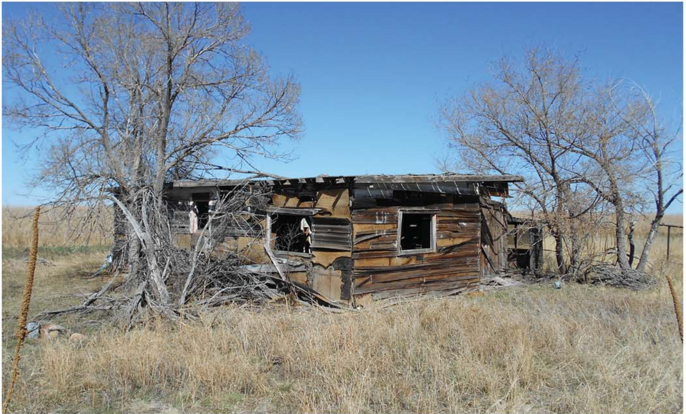
5AH3452_1: View northeast toward front side of the house.
