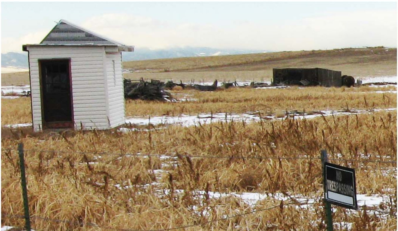
5AH3453_4: View northwest toward smaller of the two buildings. This building is located 325 feet east of larger "First Research Building" and is in close proximity to E 6th Avenue.
