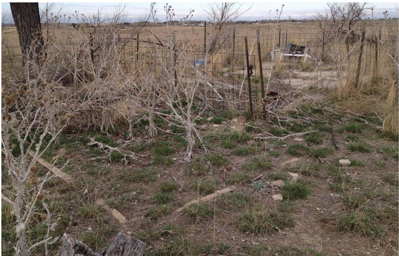
5AH3451_2: View northwest showing the south end of the concrete foundation
