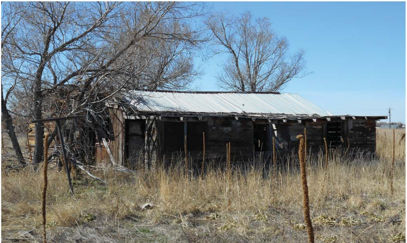
5AH3452_2: View northwest toward back side of the house.
