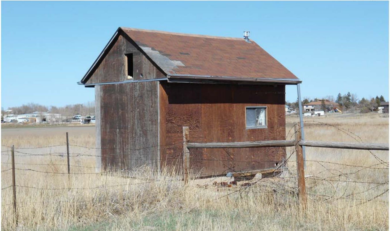
5AH3453_3: View northeast showing west elevation of "First Research Building" near west property line.
