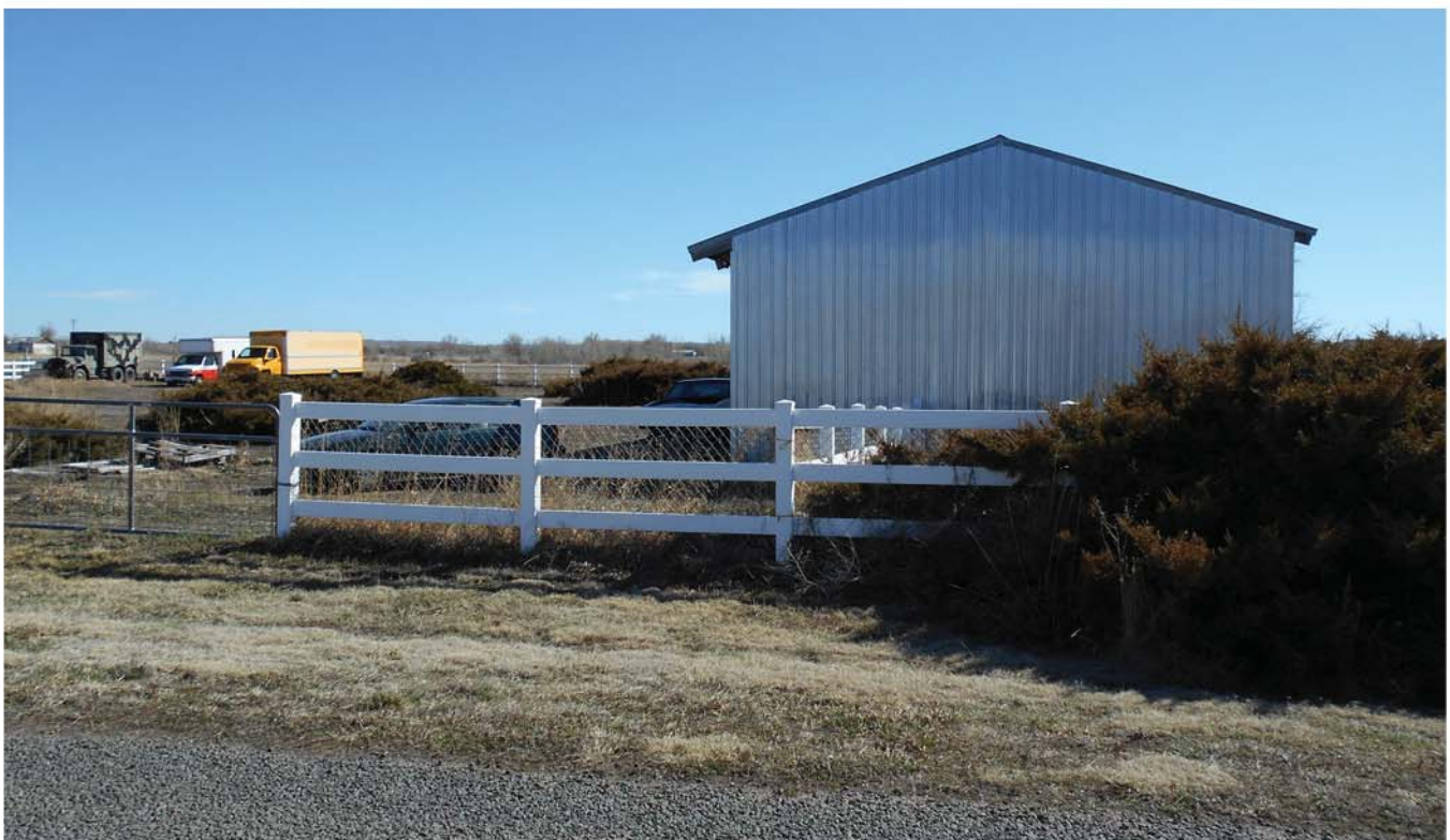
5AH3455_4: View south from E. 6th Avenue toward large metal barn at west end of property.
