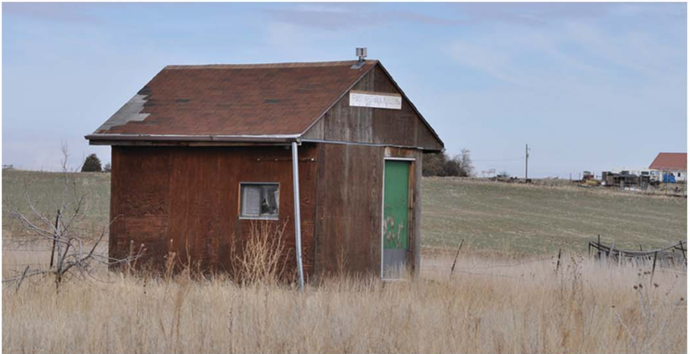
5AH3453_1: View northwest from E. 6th Avenue toward larger of the two buildings located on Project Area Parcel 115. This building is located near the west property line with a sign identifying it as "First Research Building".
